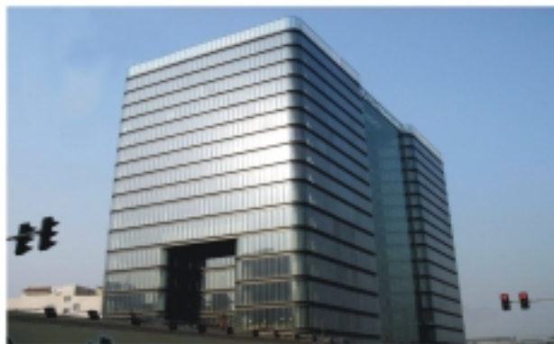
Beijing Culture Commercial Building
